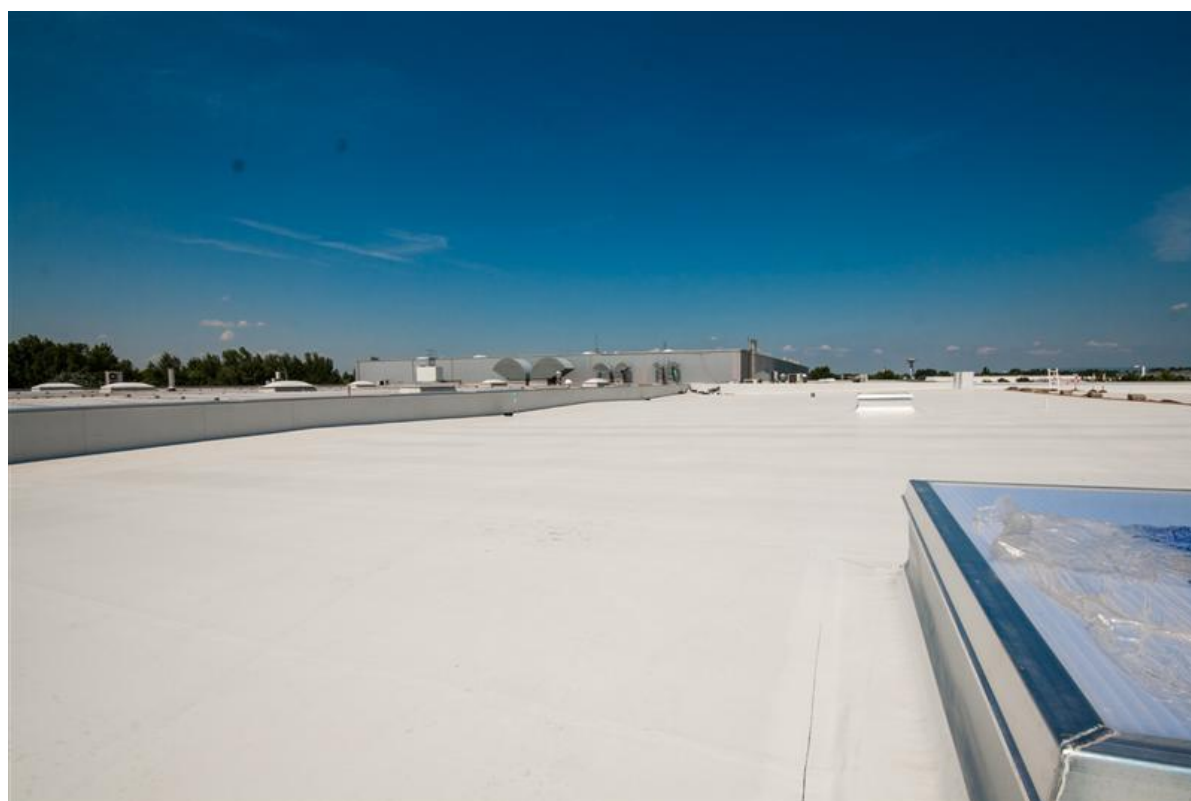
Figure 3: MAPEPLAN M on fully exposed roof
