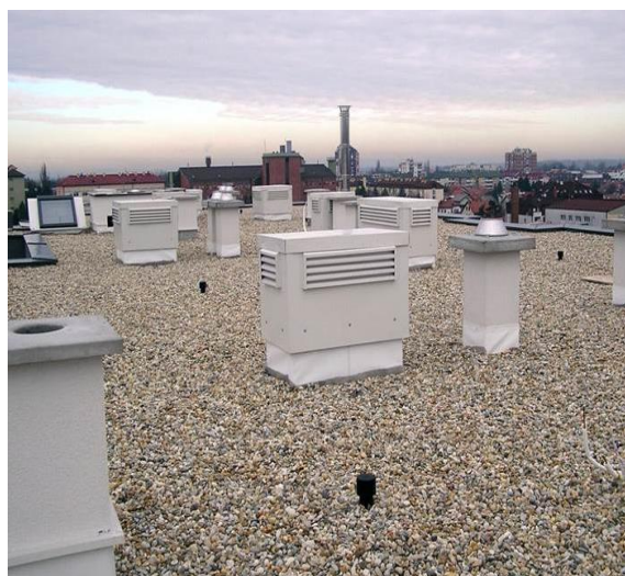
Figure 6: Membrane MAPEPLAN B on ballasted roof
