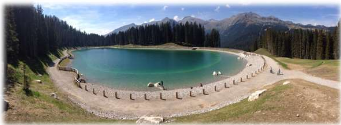
Figure 5: Membrane MAPEPLAN T WT on water reservoir
