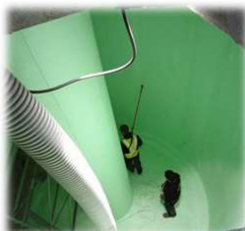
Figure 7: Membrane MAPEPLAN T WT installed on water tank
