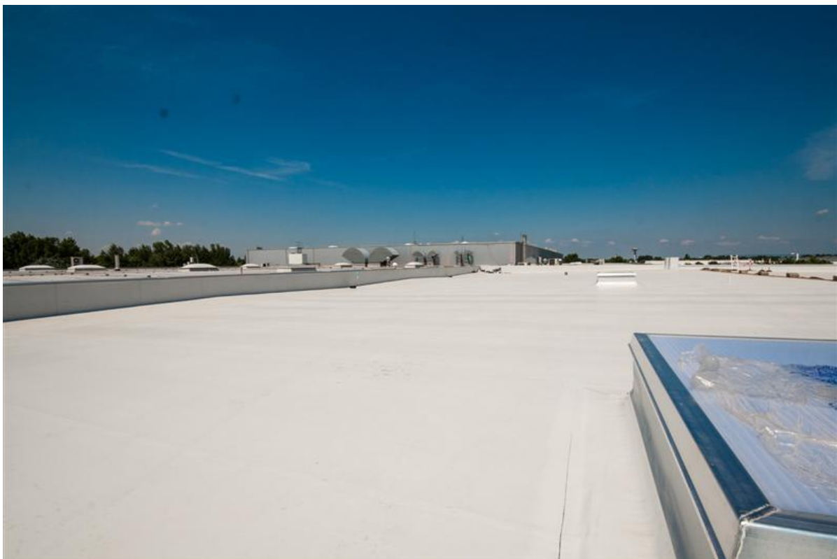
Figure 3: MAPEPLAN M on fully exposed roof
