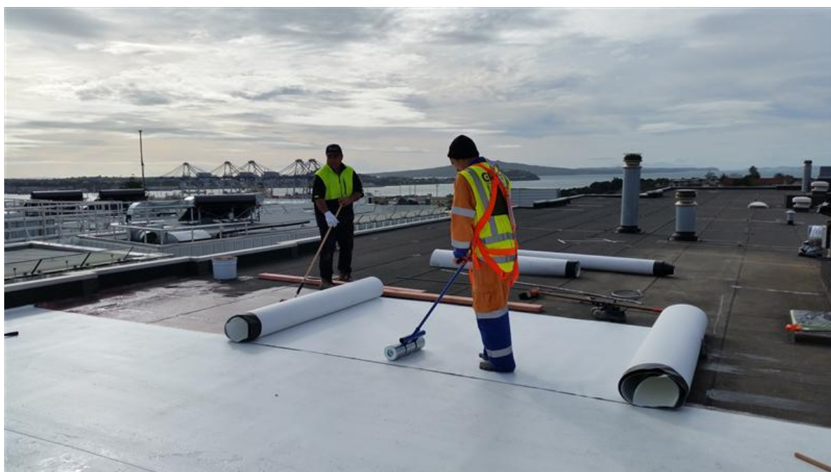
Figure 3: Membrane MAPEPLAN T Af on fully exposed roof
